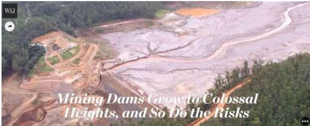
Watch the video: Massive tailings dams, like this functional one near Antonio Pereira, Brazil, are built to hold back the sludge left behind when a mill separates metals from ore. But the dams fail often enough that industry engineers are sounding alarms. Photo: João Pina for The Wall Street Journal
